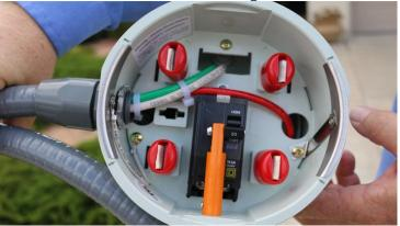
The Renewable Meter Adapter was invented to overcome a growing obstacle on the pathway to private solar–electrical panel upgrades. Typically, homes built before 1995—or nearly three quarters of American homes—require electric panel upgrades before connecting private solar. These upgrades, which can cost up to \$10,000, often include construction to walls, stucco and landscaping, introducing additional delays and permitting requirements.
